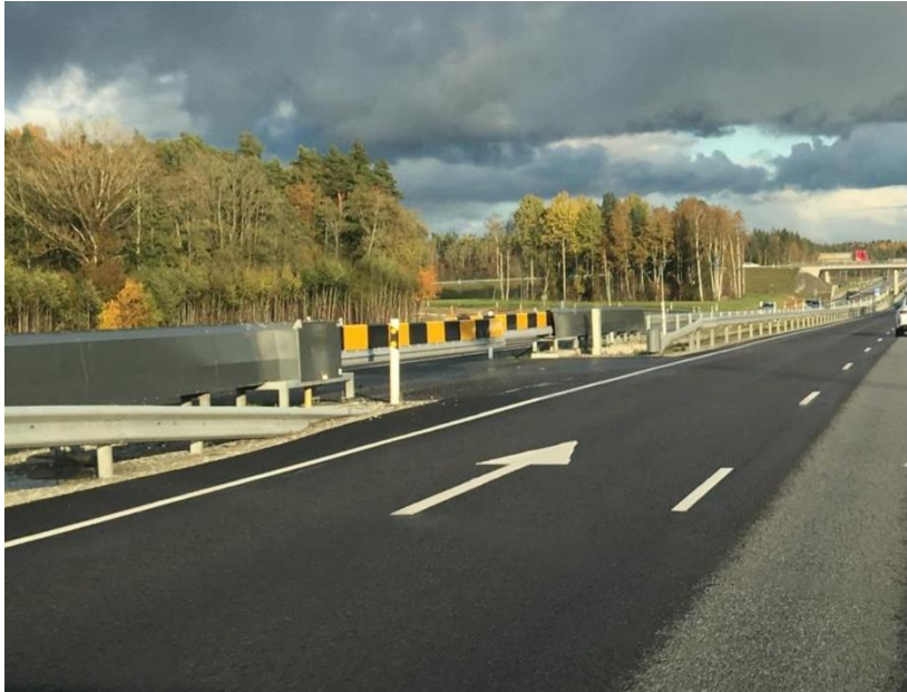
Figure 3.10 The sliding gate system in the Juuliku traffic junction
