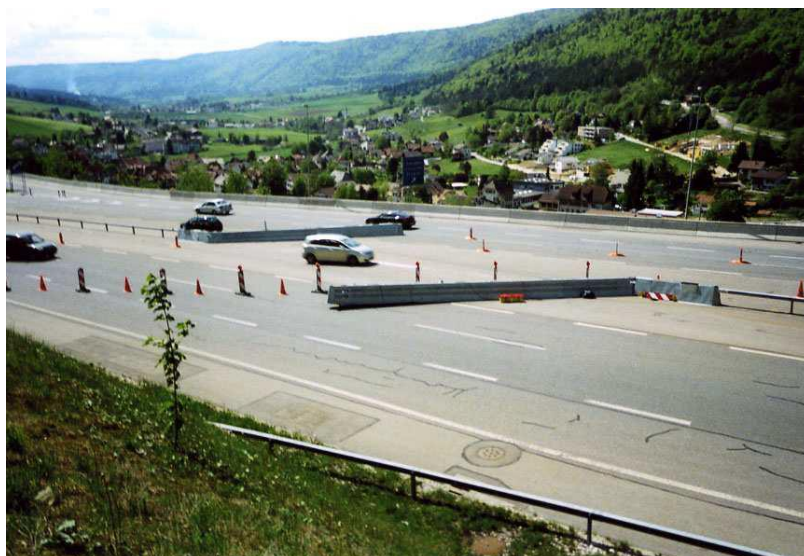
Figure 3.12 A side-opening gate system by the French company Aximum
