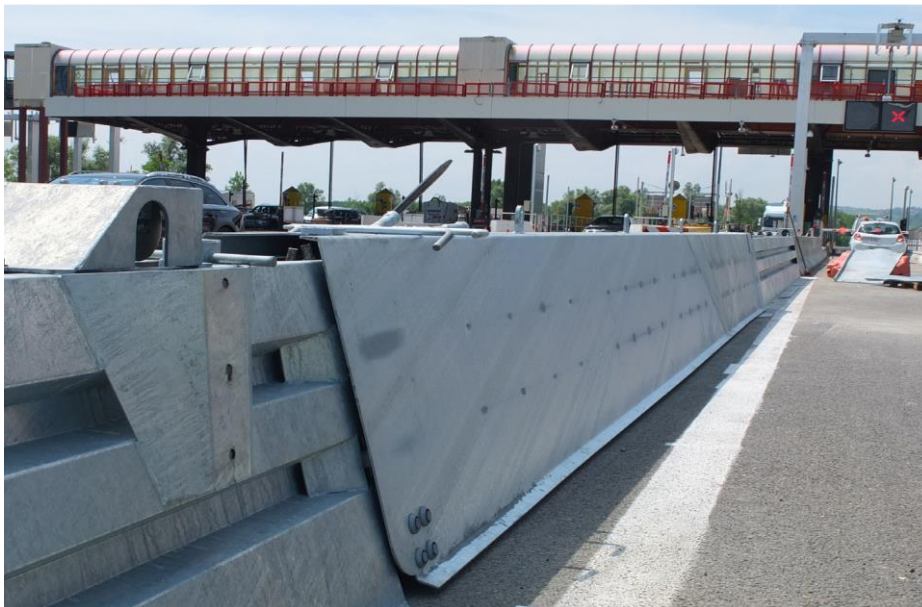
Figure 3.11 A sliding gate system of the French manufacturer Aximum which has been tested based on the requirements of EN1317.
