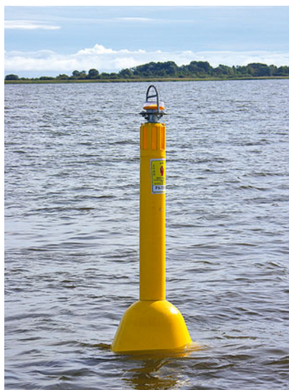
Tooder 225-1,5A laternaga Carmanah M660 Foto: Tarmo Rosenberg
