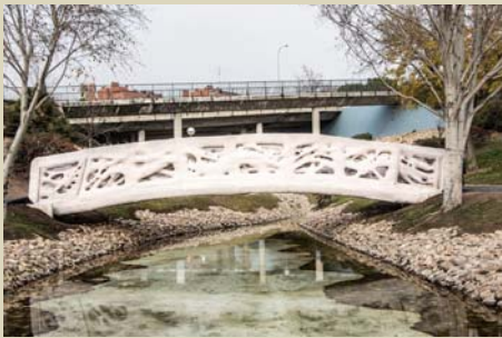
Foto: Institute for Advanced Architecture of Catalonia
