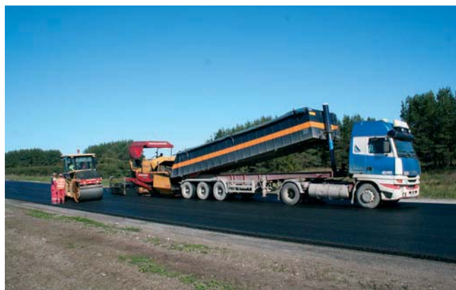
Asfaltbetoonkatte ehitamine.
