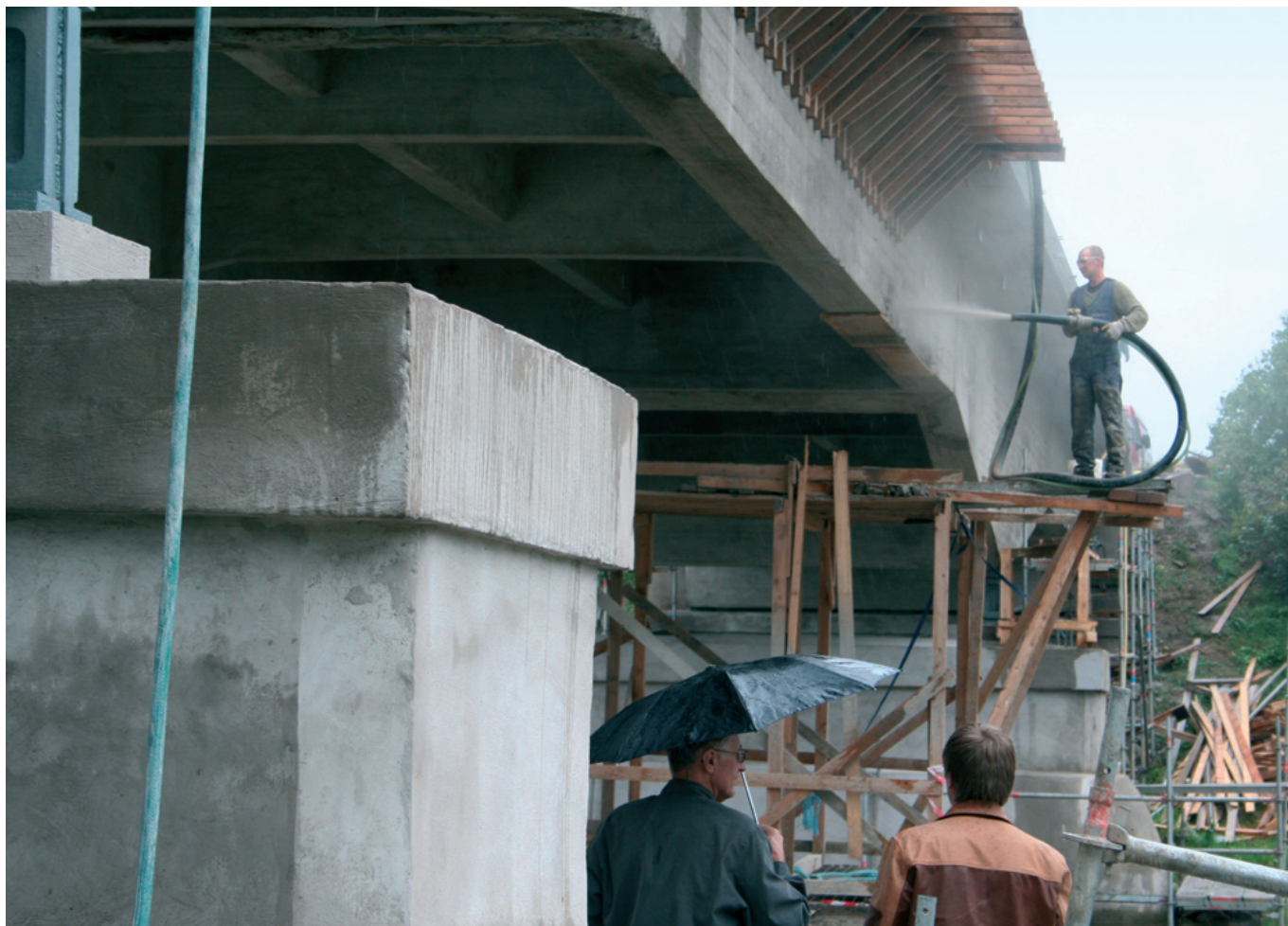
Betooni remont pritsbetooniga
