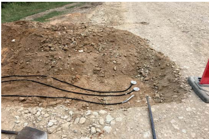
Surveandurite paigaldamine.
